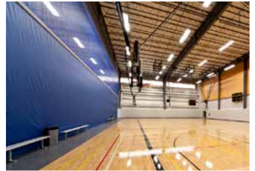
DIVIDER CURTAIN REPAIR
